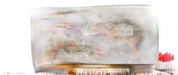
New National Art Museum of China, Beijing, (Architect: Jean Nouvel, 2014, under construction)
